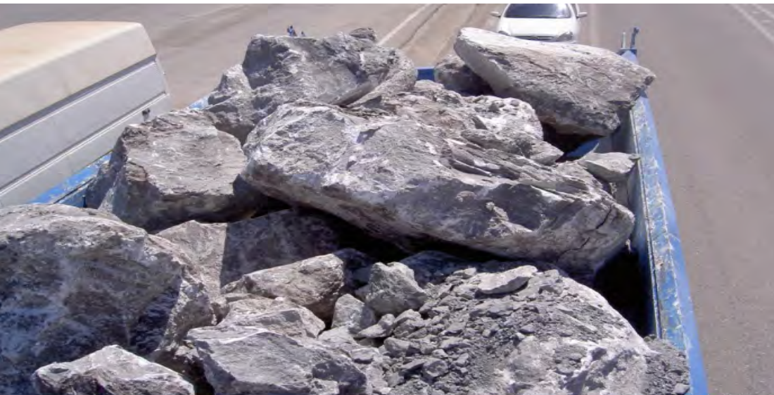
Carrying rocks for breakwater.
